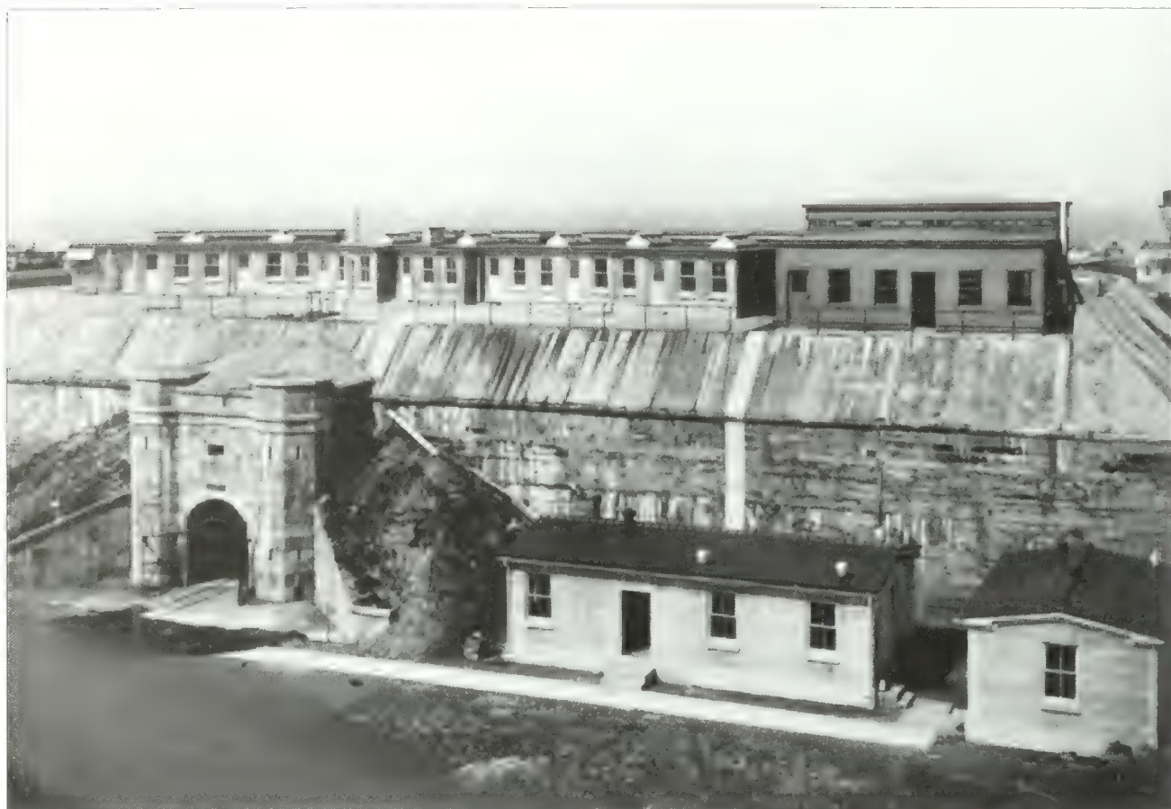
Figure 2.30. West facade of Battery Potter showing switchboard rooms, circa 1907. In order to support the communications between the fire control buildings and various batteries, the Army built two switchboard rooms at the southwest corner of Battery Potter in 1907. The two buildings required further removal of the engineered earthwork along the battery's west facade (GATE 7814).
